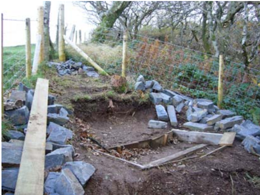
Foundations for wall and bench
